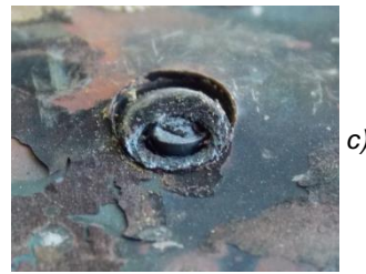
Fig. 8. Macrographic surface of rupture of the riveted tubular part. Shear test temperature of: a) 400 °C, b) 600 °C, c) 800 °C
